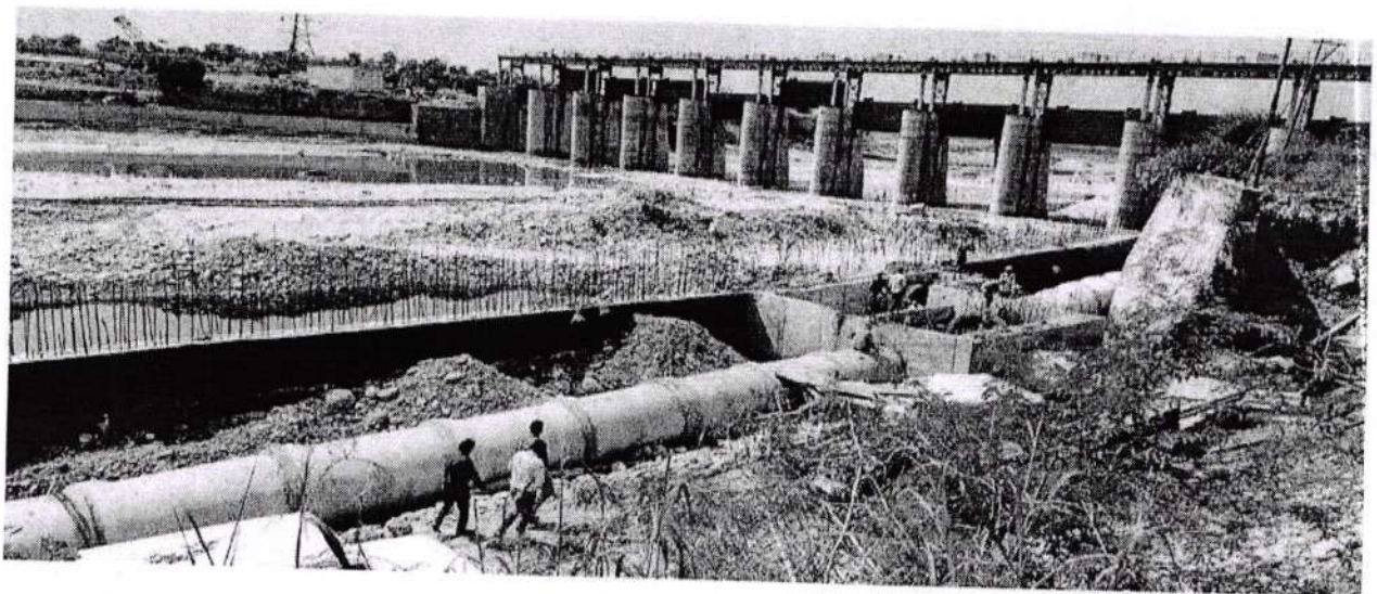
Picture showing Interceptor Drain On Right Bank
